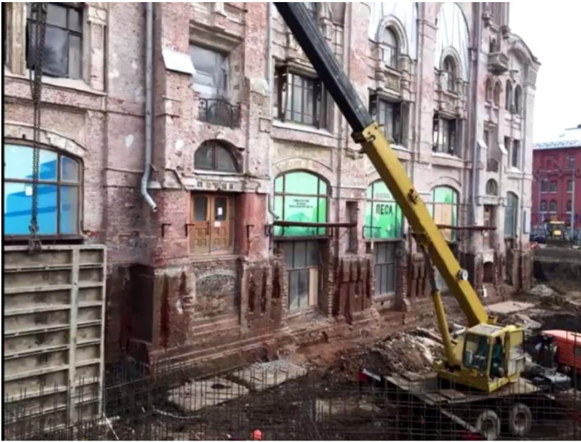
Many buildings still standing providing evidence of this cataclysm with lower floors buried in the 'Mud Flood'
